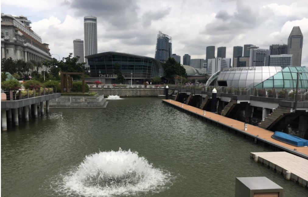
Figure 14: Marina Bay Waterfront Infrastructure
