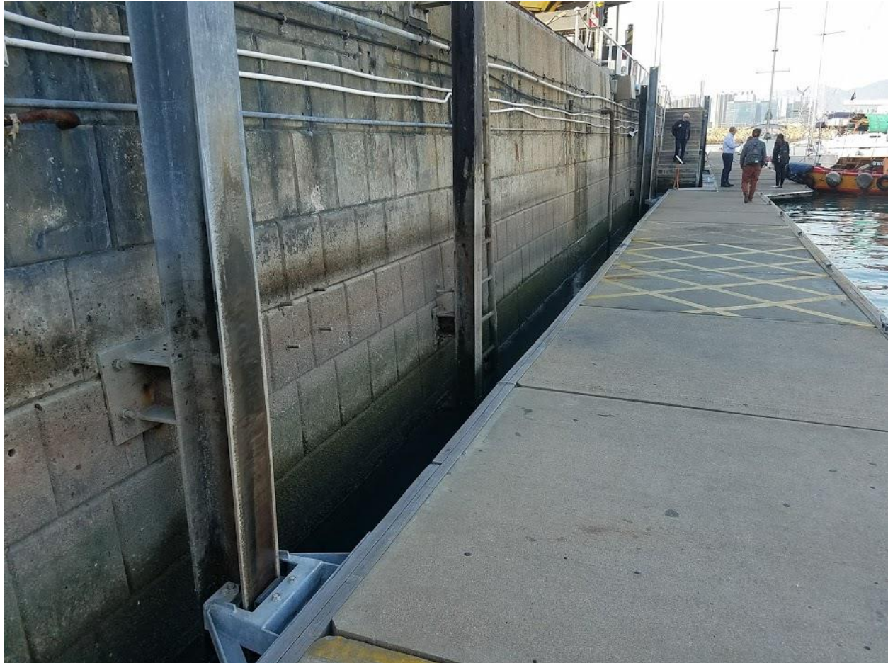
Figure D-7: Fringing pontoons operated by the RHKYC
