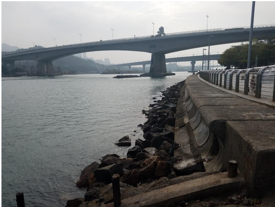
Figure D-3: Sloped Seawall with Recurve and Rubble Mound Seawall in Tsing Yi
