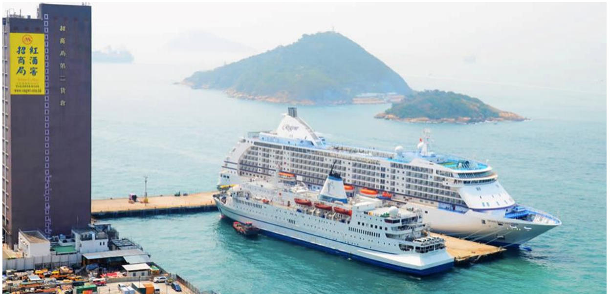
Figure 22: China Merchants Wharf Pier Future Plan (China Merchants Godown, Wharf & Transportation Co., Ltd., 2017)
