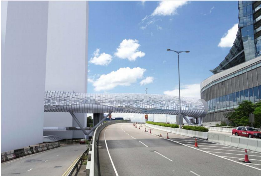
Figure F-29: Artist Square Bridge Connecting the ASDA and MTR Kowloon Station (West Kowloon Cultural District Authority, 2016)
