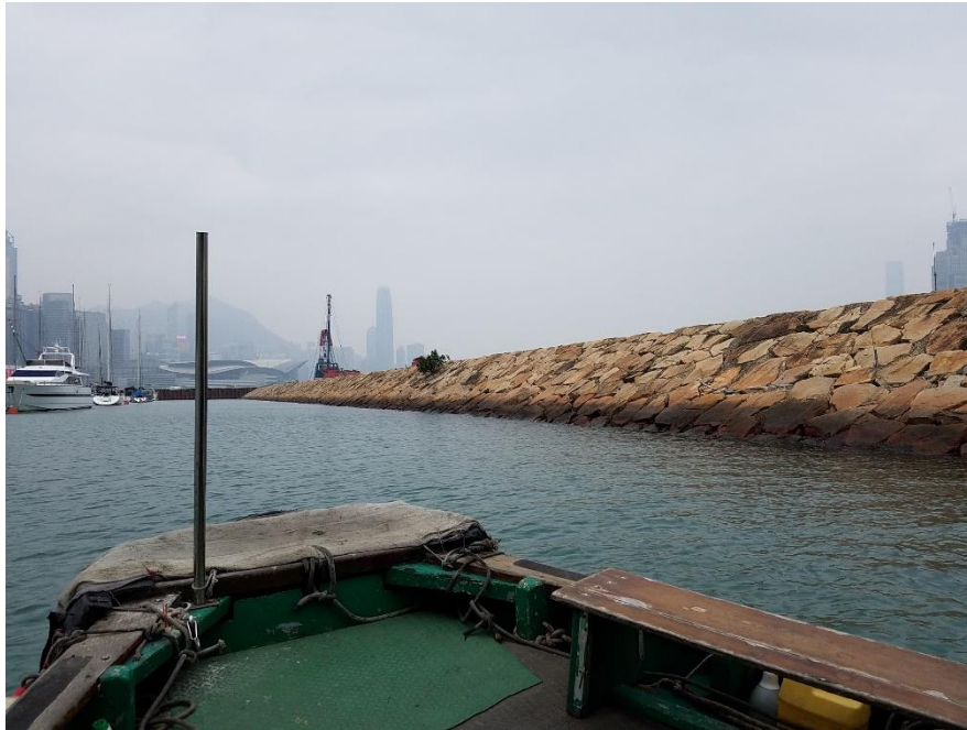
Figure F-13: Causeway Bay Typhoon Shelter Round Mound Breakwater
