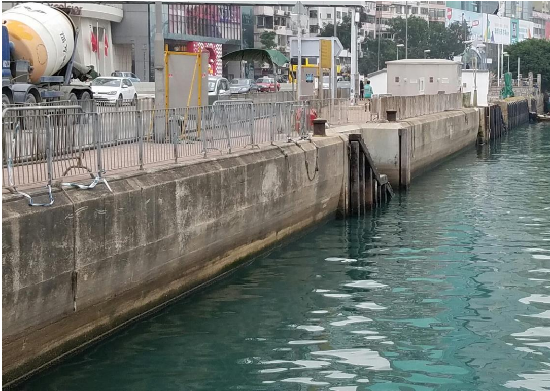
Figure D-4: Vertical Seawall in the Causeway Bay Typhoon Shelter
