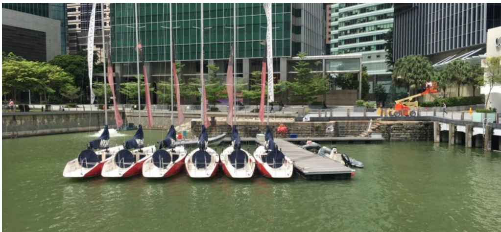
Figure 13: Marina Bay Infrastructure
