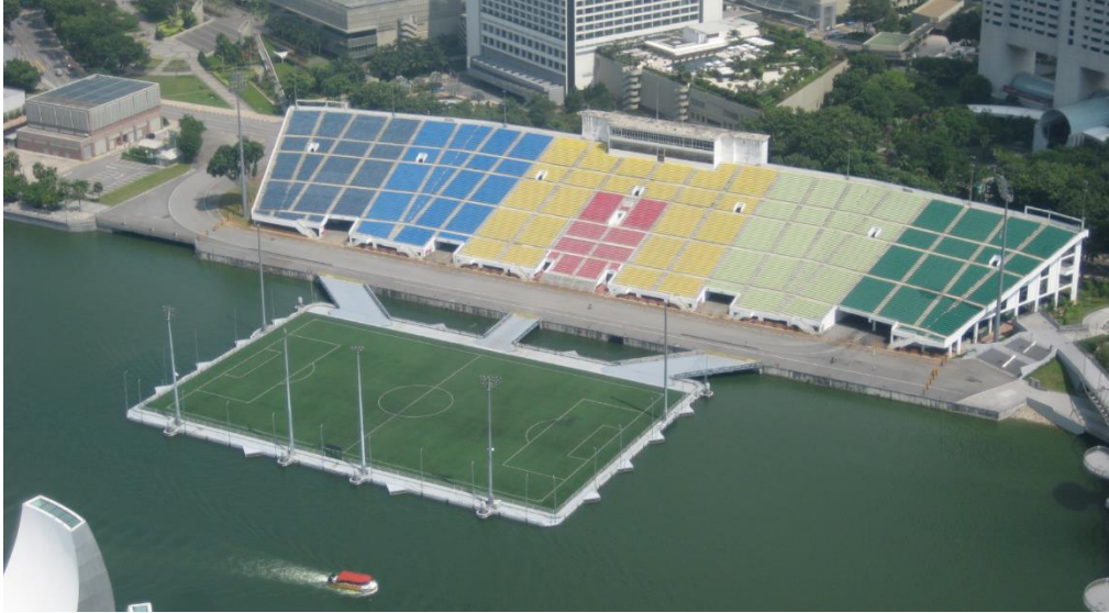
Figure 12: Marina bay floating pontoon and grandstands (Marina Bay Street Circuit Grandstand, 2012)
