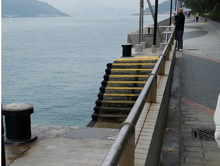
Quarry Bay Promenade Landing Step
