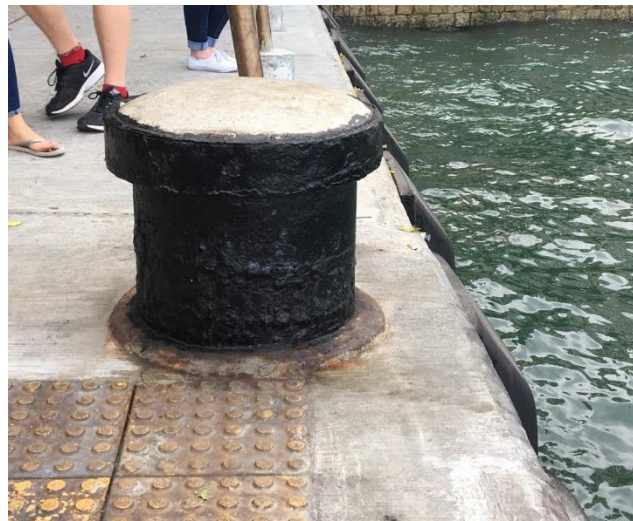
Figure D-6: Bollard along Central and Western District Promenade
