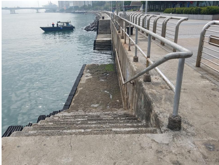
Figure D-8: Landing Steps Along the Tsing Yi Promenade
