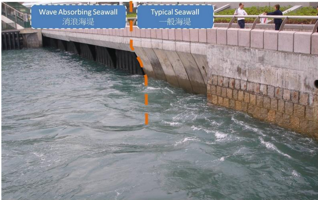
Figure D-5: The wave absorbing seawall constructed at the harbour-front near the Central Piers (CEDD, 2012)
